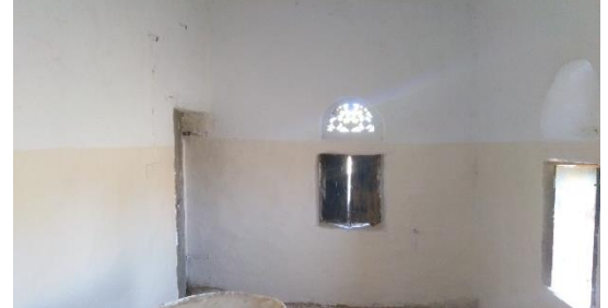
Before and after the repainting of the interior
