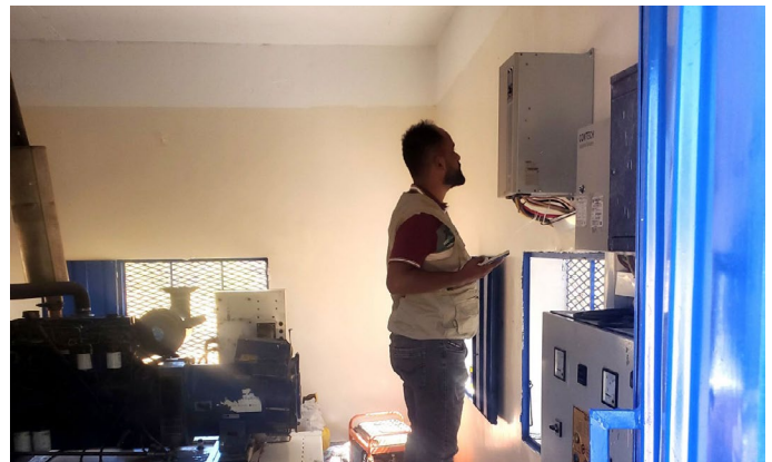
YFCA worker while installing the solar energy inverter.
