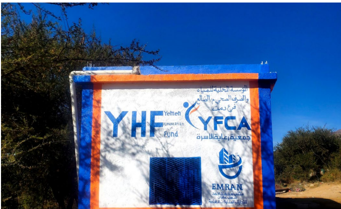
The well after the complete rehabilitation intervention.
