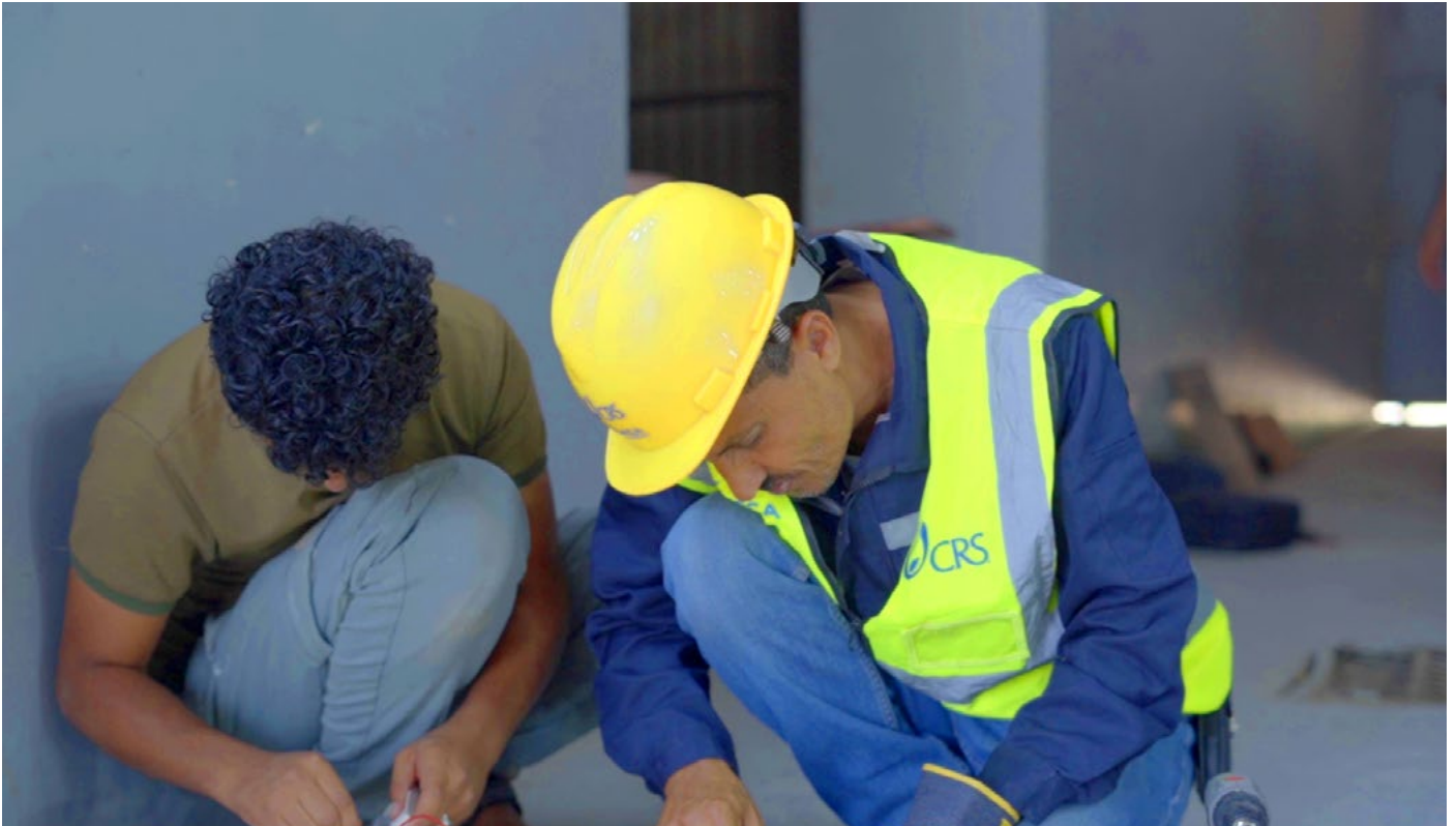
Shahim practices assembling and wiring electrical junction boxes during practical training.
