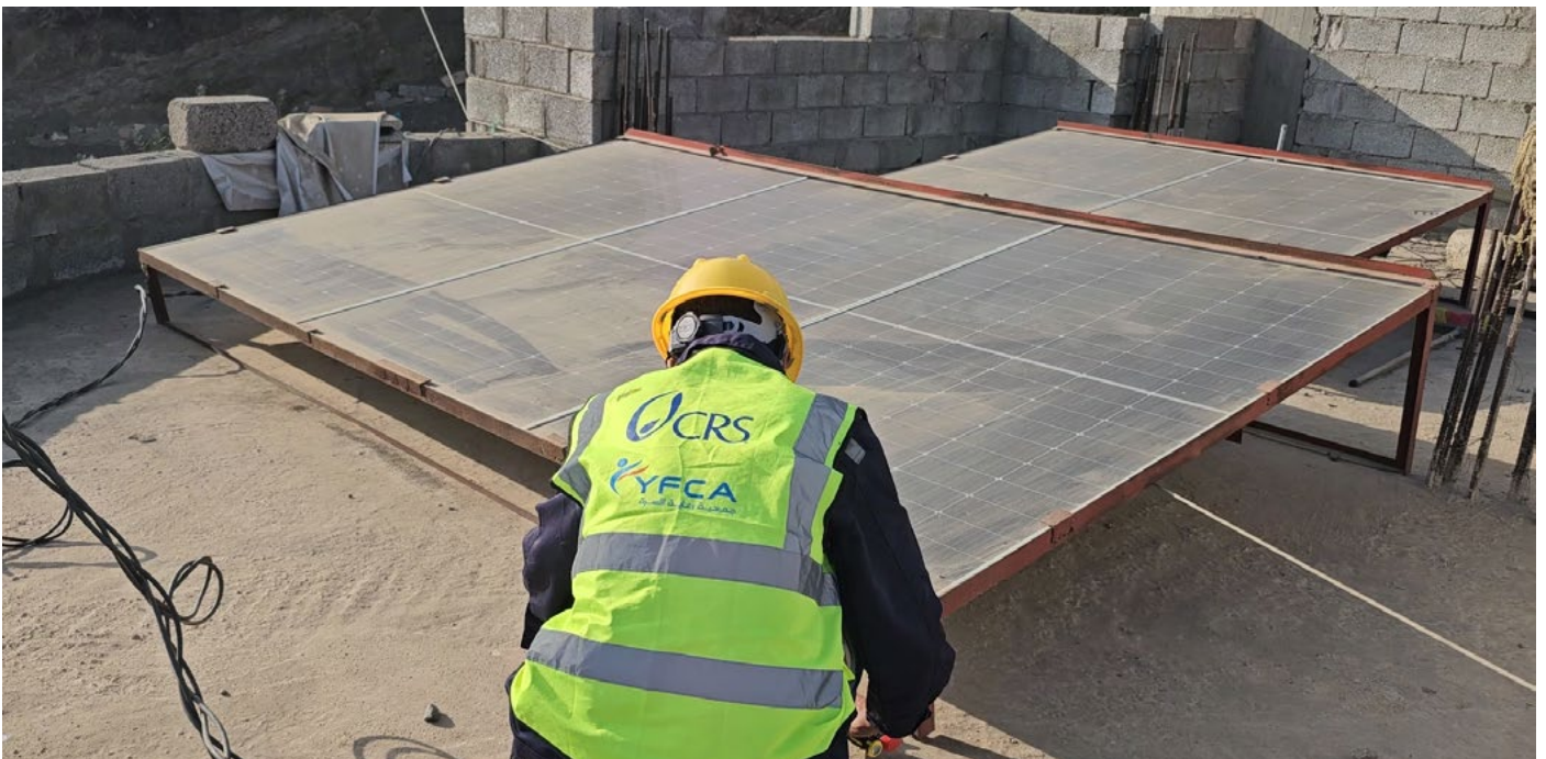
Shahim inspects and adjusts ground-mounted solar panel frameworks on a rooftop as part of his technical installation services.
