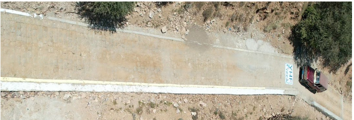
The road after being fully paved.
