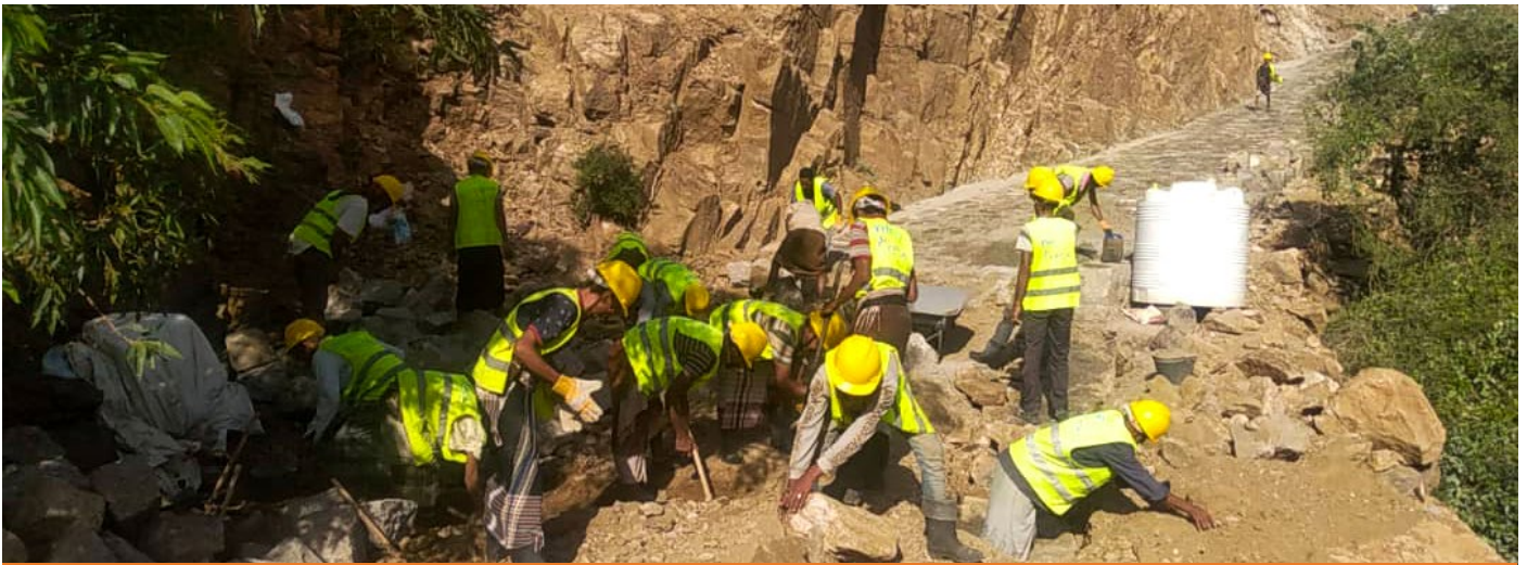
CFW workers during paving the road.
