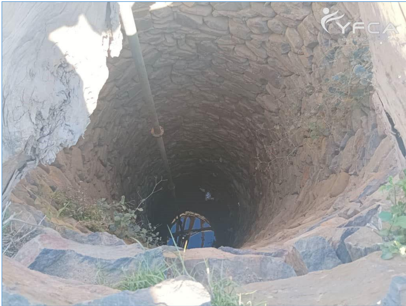
Photo 8 An Unprotected Well _ Jayshan District
